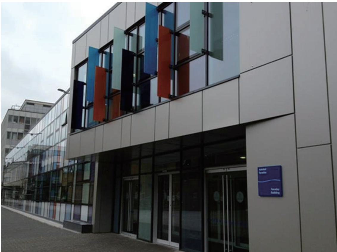
1) Faraday building outside
